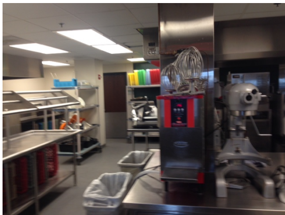
Figure D.3: Penthouse Kitchen
