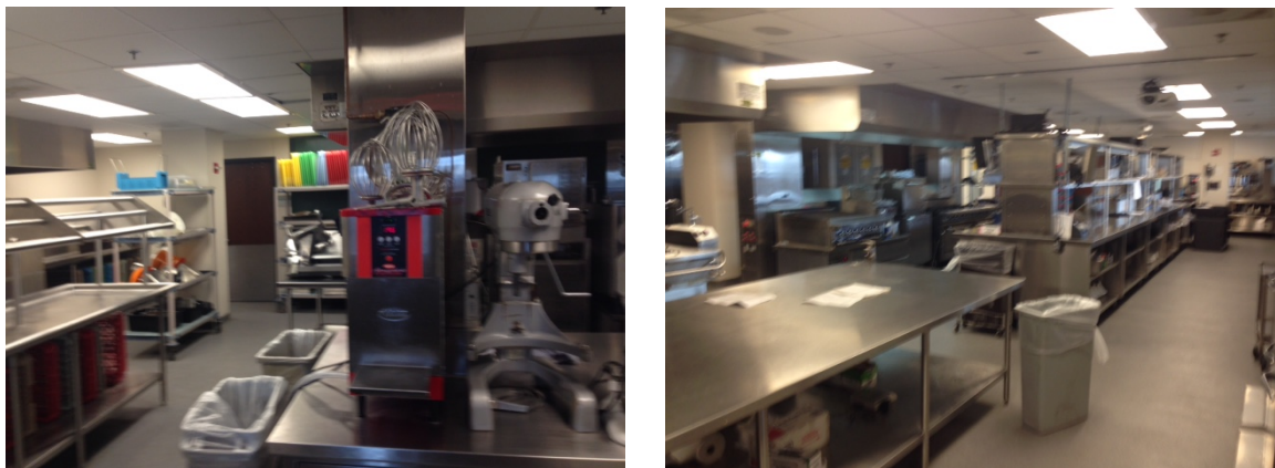
Figure D.3: Penthouse Kitchen
